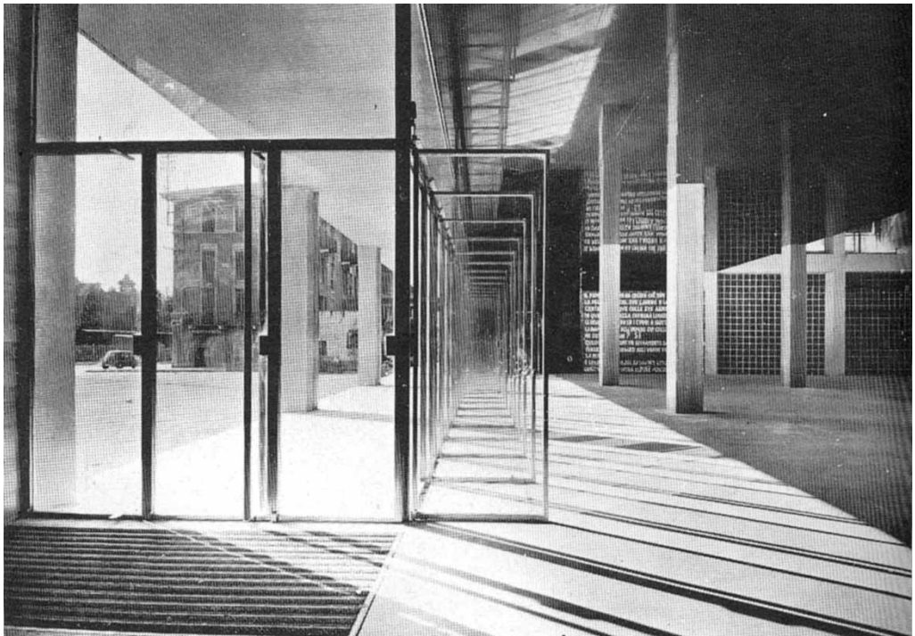
Figure 6. Giuseppe Terragni, Casa del Fascio, Como, 1936: the entry doors seen in file. (Courtesy of the Centro Studi Giuseppe Terragni, Como.)
